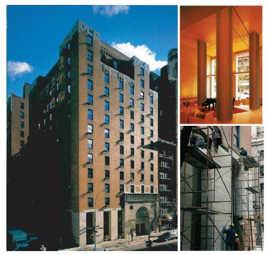
*Clockwise from top: Completed exterior restoration of the Roger Williams Hotel. The finely honed, limestone interior walls of the grand lobby. Urban D.C.'s in-house crew, installing the structural steel that supports the window openings.*
