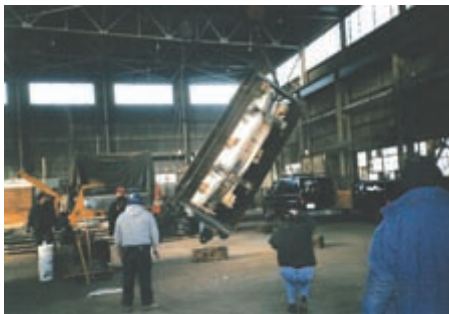
Photo above: Detail of mosaic after the completion of full resetting and reinstallation. Photo bottom left: Urban D.C.'s in-house crew flips the precious mosaic to begin structural work. Photo bottom right: Urban D.C. setting the structural steel into mosaic's underside.
