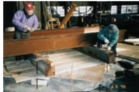
Photo above: Detail of mosaic after the completion of full resetting and reinstallation. Photo bottom left: Urban D.C.'s in-house crew flips the precious mosaic to begin structural work. Photo bottom right: Urban D.C. setting the structural steel into mosaic's underside.
